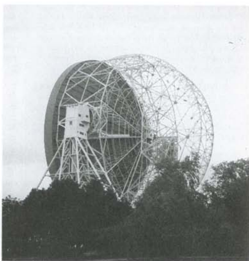
The 76m dish at Jodrell Bank. Two large wheels stabilize the rear of the dish and provide elevation control, and the whole enormous thing rotates in azimuth on a railway track.
